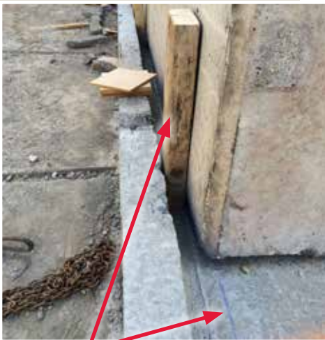
2"x4's and chalked line are used for alignment.
