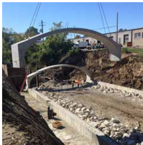
Second unit is lowered into place.
