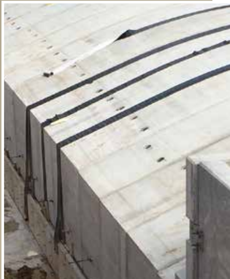
Joint wrap in progress.
