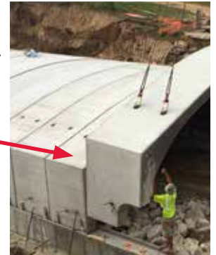
Tip units slightly for easier fit.
