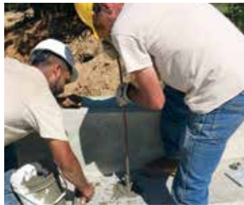
Grouting the bolts of the headwall.
