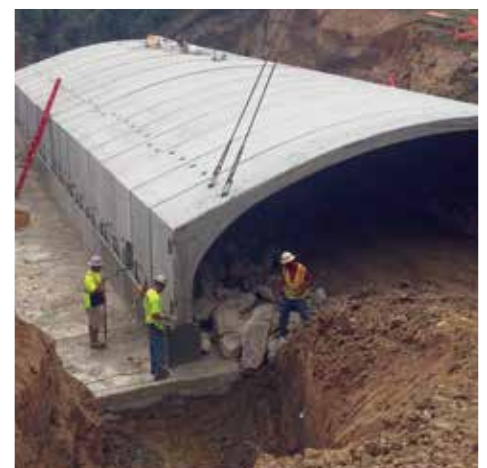
Last unit is set, before setting the headwalls and wingwalls.
