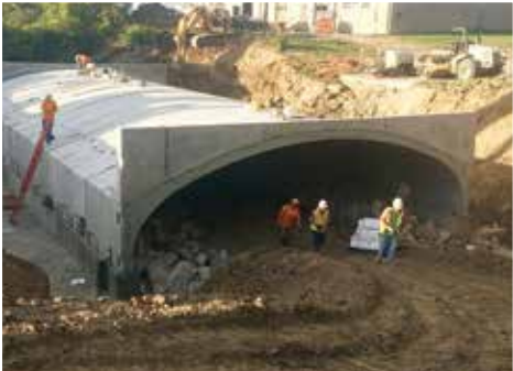
The finished headwall.
