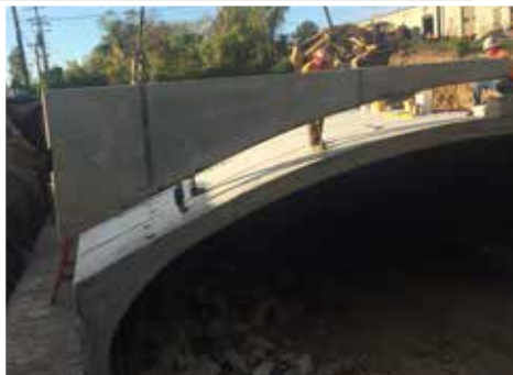
Headwall unit is moved into position.
