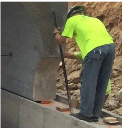
Shim pads are used to control elevation.
