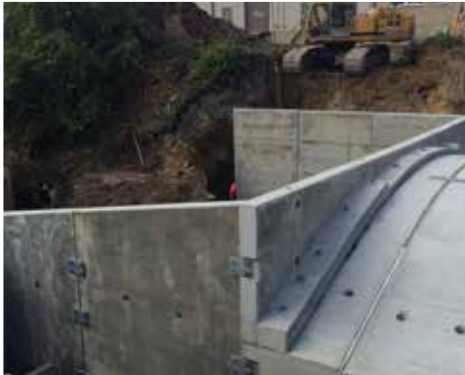
Bolted plates are shown attached.
