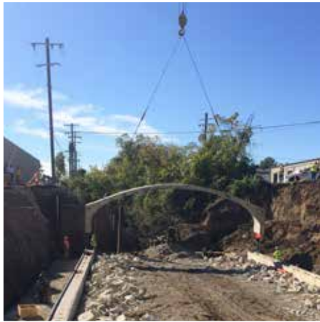
First unit being set.
