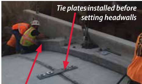
Headwall units are bolted into place.
