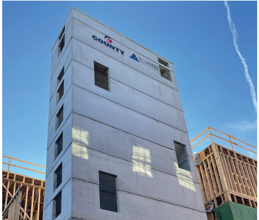
Four Story Stair Shaft
