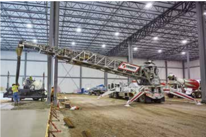
Telebelt Material Conveyor
