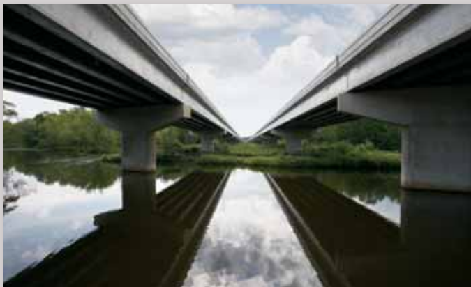
Hwy 10 Bridge Crossing
