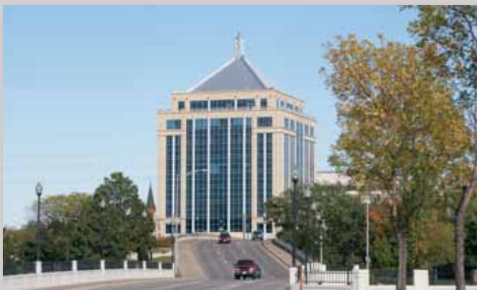
First Wausau Towers-Dudley Building
