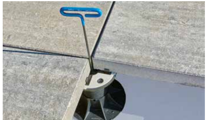
Easy adjustment with pavers in place
