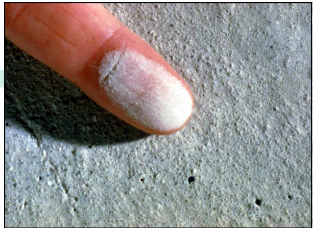
Dusting concrete surface
