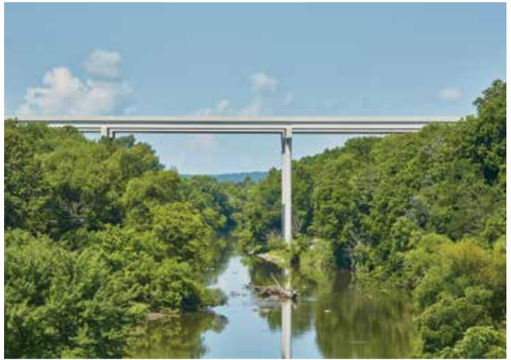
*Spanning over the Baraboo River, two 160-foot-tall concrete prestress bridges were constructed along U.S. 12, making them the tallest bridges in Wisconsin.*
