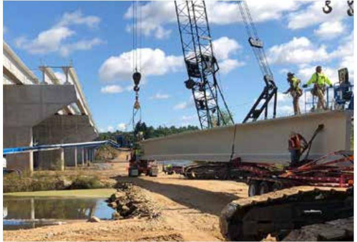
Girder delivery and installation had to be precisely timed and coordinated to accommodate fluctuating river water levels that were impacted by rain events. County Materials' dispatch team and heavy haul truck drivers from both the Janesville, WI and Roberts, WI locations worked in tandem with the construction teams onsite to ensure effective communication and to meet project timelines. The bridge officially opened for traffic at the end of 2019.
