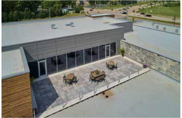
Skylands Concrete Deck Pavers are installed on a pedestal system that is designed to transform underutilized spaces. These systems accommodate a range of slopes for diverse applications. Using a pedestal system, pavers are installed evenly to promote proper drainage through joints, preventing puddling and improving pedestrian safety. Once installed, the complete system protects the roof below from seasonal elements while ensuring easy maintenance access.
