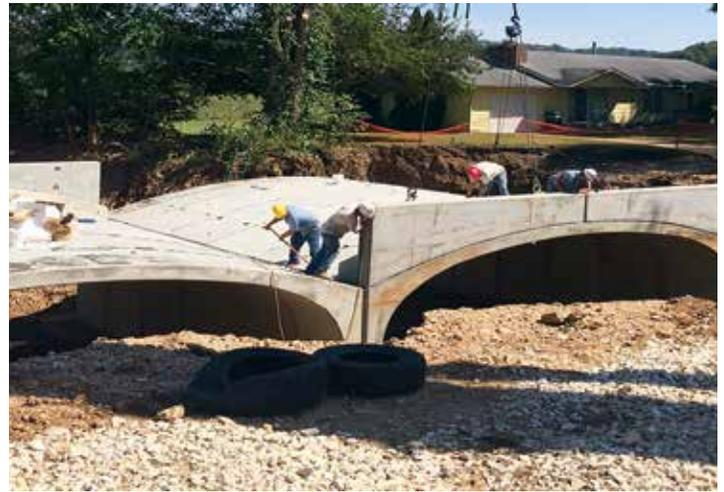
The city selected County Materials' ArchCast bridge system for its highly durable and straightforward three-sided design. County Materials manufactures the system and delivers the product to the site ready for quick installation. Additionally, because of budget constraints, city officials decided the best option for saving costs was to build the bridge using their crews, without hiring any outside contractor.
