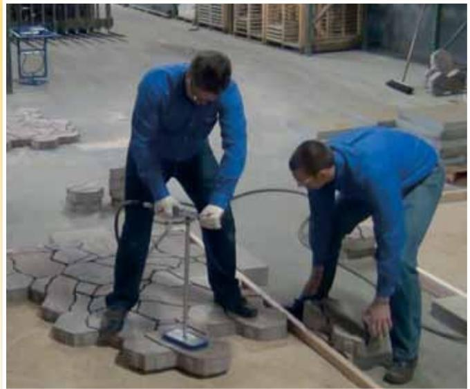
*The use of paver installation equipment, such as a one-person (shown above) or two-person pneumatic handling unit, makes it easy to maneuver random size pavers and larger slabs, and install more square footage in less time.*
